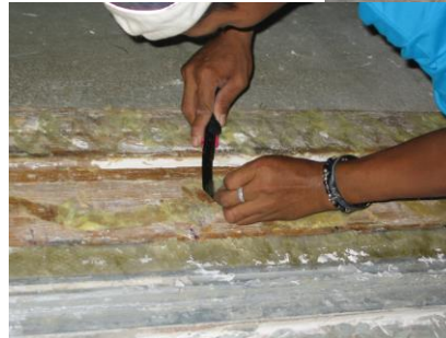
Repairing the Isolation joint between chambers before tests.
