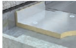
Typical Installation - Concrete Deck
